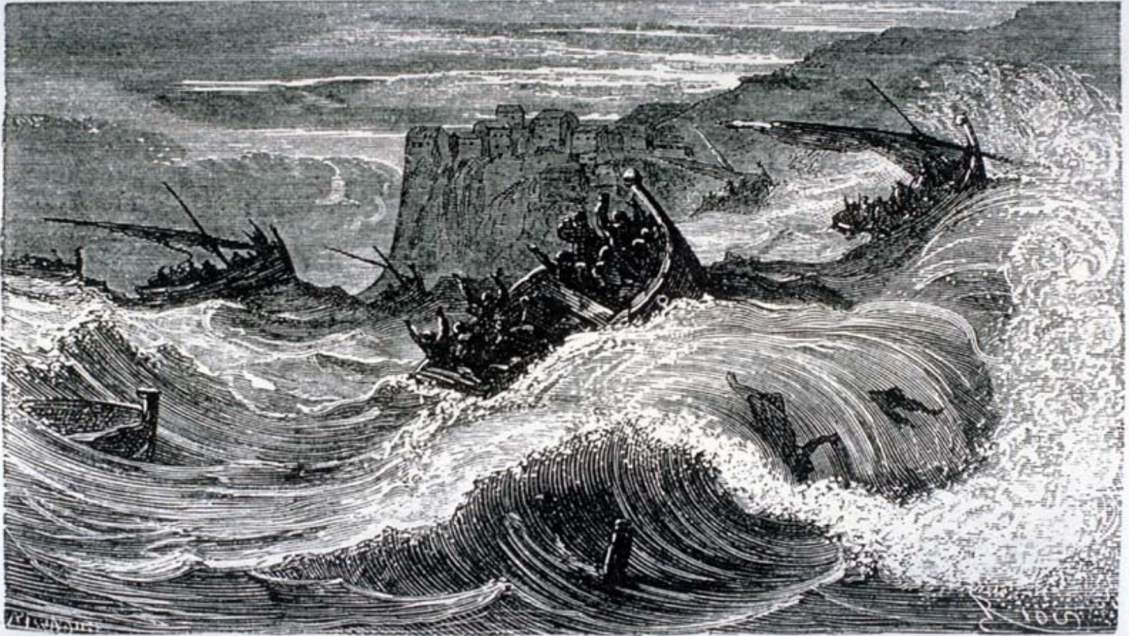
Fig. 55. —INCIDENT DURING THE EARTHQUAKE AT SUMATRA (1861).
